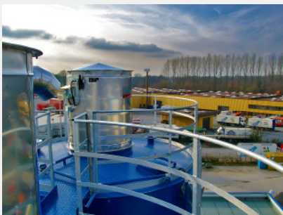
View from the silo bunker to the residual area
