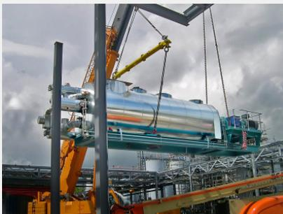
Installation of the dryer unit
